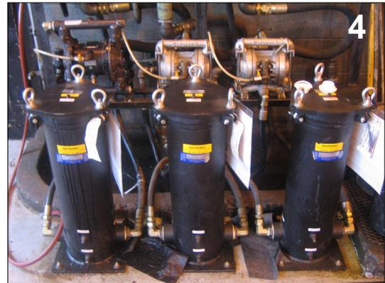
Hy-Dry Desiccant breathers were installed on all tanks to prevent water and particulate contaminant from entering the bulk tanks (photo 5). The Hy-Dry breathers control particulate contamination down to 4µ[c] with 99.95% efficiency. The desiccant adsorbs the water as the air entering the reservoir passes through the breather. As the breather collects water the desiccant changes color from gold to dark green which signals the need for replacement.
